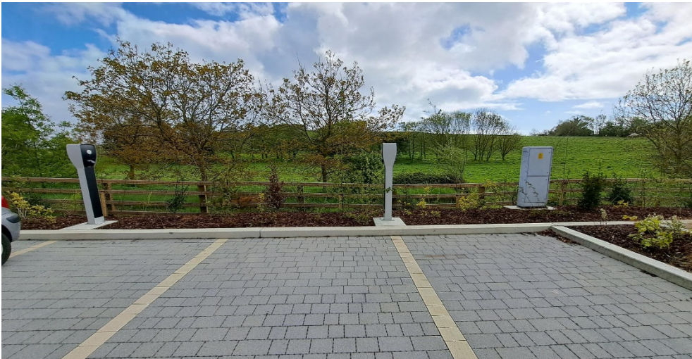
Figure 10: Typical Double head EV charging pillars and double height ESB metered pillar
