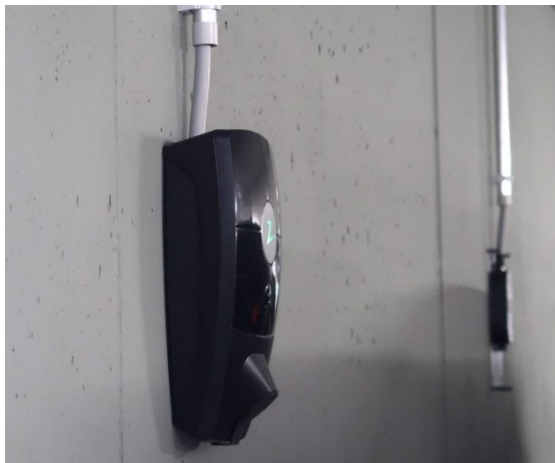
Figure 8: Typical wall mounted car domestic car charger
