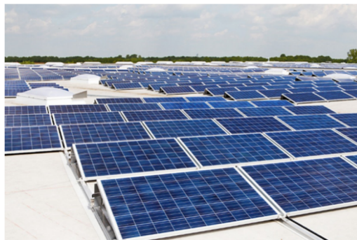
Figure 4: Photovoltaic Panels Example
